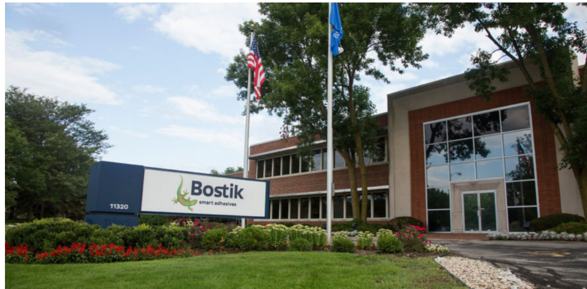
Bostik Center of Excellence for Hot Melt Technologies in Wauwatosa, Wisconsin
