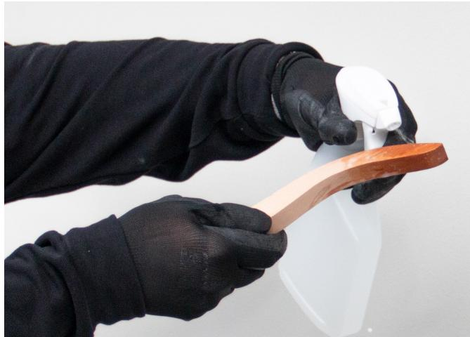
Use Finisher and a wooden spatula to tool the fresh joint. Only wet the spatula with Finisher. Do not spray directly onto the fresh sealant.
