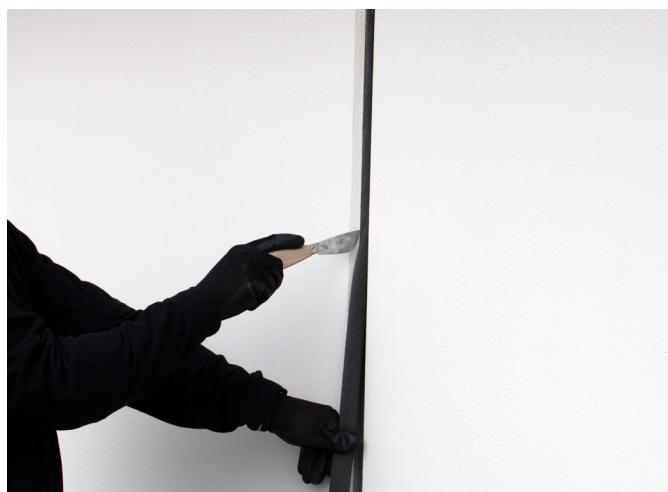
Apply the Backer Rod at the right depth. Make sure that the size of the Backer Rod is 150% of the width of the joint.
