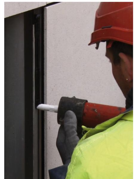
use thinner panels and lighter support structures. Bonded panels also withstand vibration better than mechanically fastened panels.
