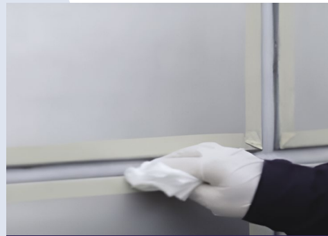
Using Bostik Primer (if necessary) by two way cloth method
