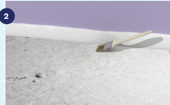
STEP 2. Apply Bostik Liquid Waterproofing Membrane by brush, roller or trowel to the joints between wall and floors and vertical wall-to-wall joints paying particular attention to corners.
