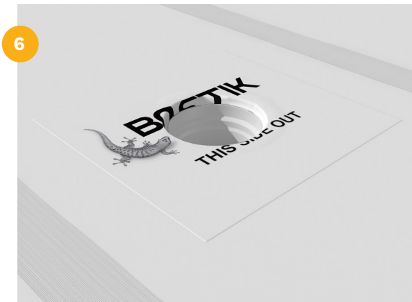
6 Remove the mounting jig and mold the foil and drain seal so it touches the inside edge of the well.
