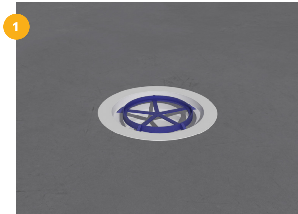
1 Make sure the floor is clean and free of dust.
