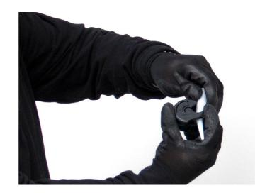
Cut the cartridge nozzle at a 30 degree angle and at Apply the sealant at a steady pace and in sufficient the width that corresponds to the size of the joint. volume to fill the joint. Make sure the sealant makes contact to both adhesion surfaces.
