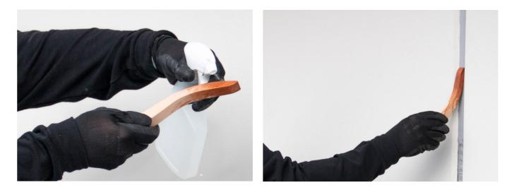
Use Finisher and a wooden spatula to tool the fresh Tool the fresh sealant joint with the wetted spatula. joint. Only wet the spatula with Finisher. Do not spray directly onto the fresh sealant.
