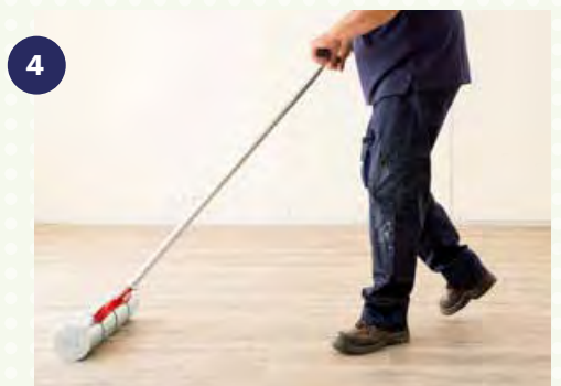
4 To ensure the perfect transfer of the adhesive and obtain the right final result, use a heavy metal roll (+/- 60 kg).
