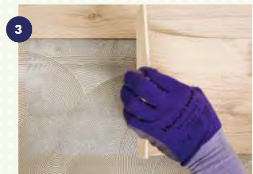
3 Lay the floor covering while the adhesive remains tacky and receptive. Wait 24 hours to achieve the curing time of the adhesive.
