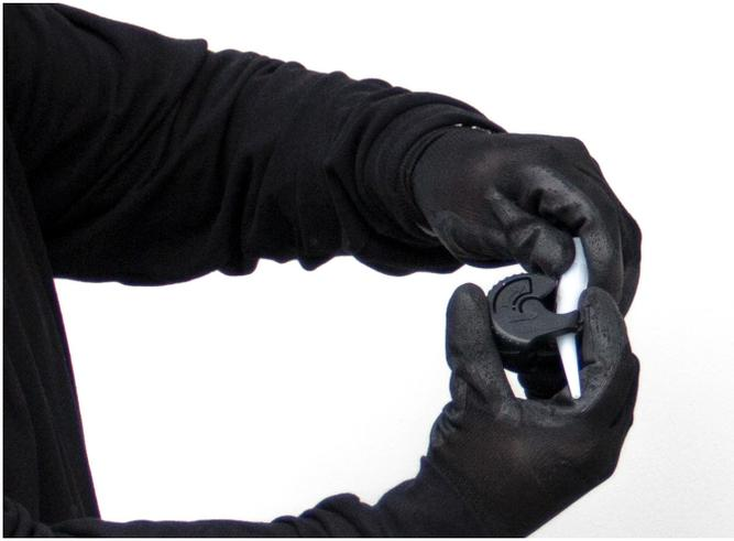
Cut the cartridge nozzle at a 30 degree angle and at the width that corresponds to the size of the joint.
