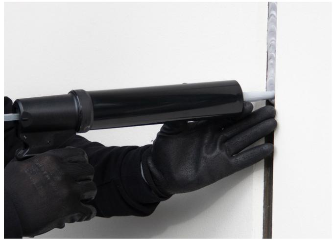
Apply the sealant at a steady pace and in sufficient volume to fill the joint. Make sure the sealant makes contact to both adhesion surfaces.
