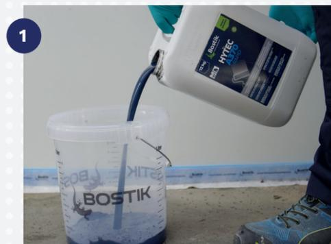
1 Pour HYTEC A370 RAPID into a **clean bucket or paint tray to facilitate the application of the medium hair roller.**
