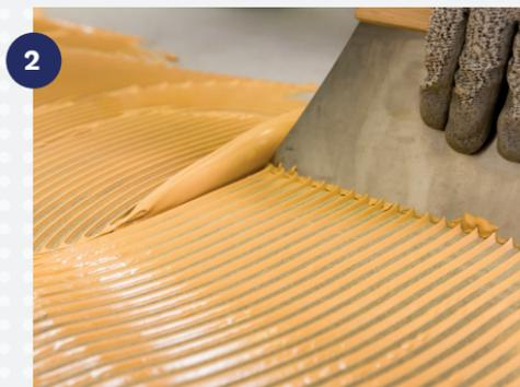
Once dried, apply the **wood floor adhesive** directly over the **HYTEC P510 RENORAPID** with the approved notched trowel **spatula TKB-B12**.
