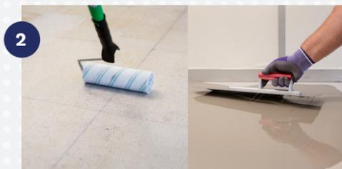
Application of **GRIP A936 XPRESS** (100g/m<sup>2</sup>) on the resin and after 2h apply the self-levelling compound over the entire surface.
