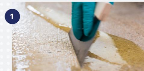
Application with a **notched trowel TKB-B2** in 2 coats at 24h intervals at a rate of 400g/m<sup>2</sup> for the 1st coat and 300g/m<sup>2</sup> for the 2nd coat.
