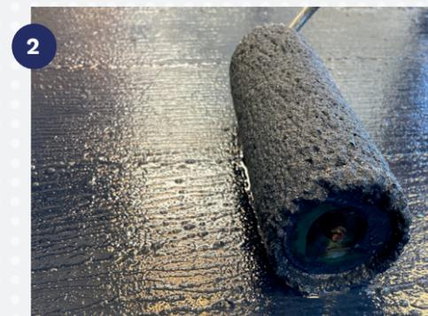
2 Apply the 1st coat of the undiluted HYTEC A370 RAPID using a medium hair roller at a rate of **150g/m<sup>2</sup>/coat.**
