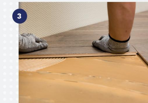
No waiting time needed, place the wood floor covering and **press firmly** to ensure a good transfer.
