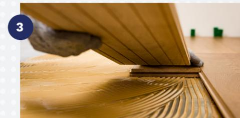
Application of the wood floor adhesive for solid parquet installation.
