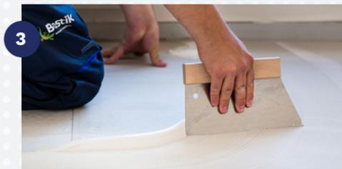
Application of the adhesive for soft floor covering installation.
