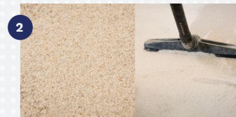
**Broadcast sand (BOSTIK S409)** in excess on the 2nd layer over the fresh resin, then vacuum the excess sand after 24h.
