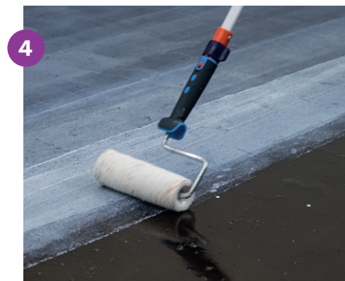
4 Apply GRIP A936 XPRESS primer with a short hair roller (100-120 g/m 2 ). Allow a drying time of 2 hours before applying the self-levelling compound.
