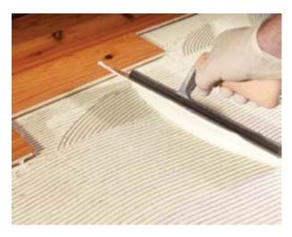
or leveling must be done using a Portland-cement-based material (e.g., Bostik Webcrete® 95, Webcrete® 98, SL-100™, SL-150™, SL-175™, SL-200™, SL-Rapid™, or UltraFinish™ Pro).
