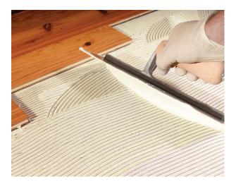
No. 03732). Maximum acceptable floor variation is 3/16" in 10 feet. Areas requiring patching or leveling must be done using a Portland cement-based material (e.g., Bostik UltraFinish<sup>™</sup> Pro, Webcrete<sup>®</sup> 95, Webcrete<sup>®</sup> 98, SL-100<sup>™</sup>, SL-150<sup>™</sup>, SL-175<sup>™</sup> or SL-200<sup>™</sup>).
