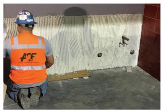
Projects calling for gauged thin porcelain tile panels now can be installed in roughly half the time with a smaller crew — only a single layer of adhesive is troweled onto the back of the panel or wall, cutting the square footage necessary to trowel in half.
