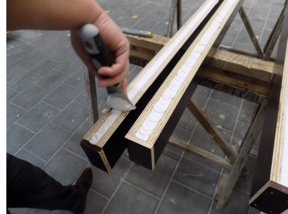
mounting of the sealant
