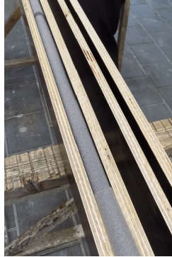
mounting of the sealant
