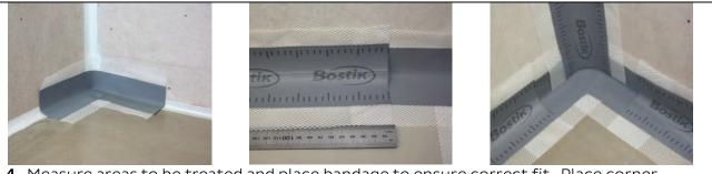
Measure areas to be treated and place bandage to ensure correct fit. Place corner section first and allow for at least 40mm overlap at all joins. Ensure that in vertical overlaps the top section of bandage is placed over the bottom section (ie flashed)
