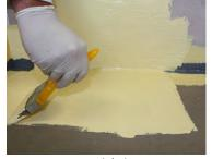
Apply first coat of membrane at correct thickness across entire section (including full surface of bandage).
