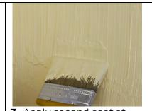
Apply second coat at correct thickness perpendicular to first.
