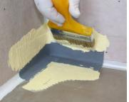
**5.** Secure bandage by applying chosen membrane to open flexible weave.
