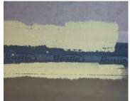
Place additional sections of bandage with sufficient overlap (min 40mm). Always place with printed face up. Secure bandage by applying chosen membrane to open flexible weave. Leave to touch dry. This is a good time to check integrity of bandage system as repairs will be more difficult after membrane is applied.
