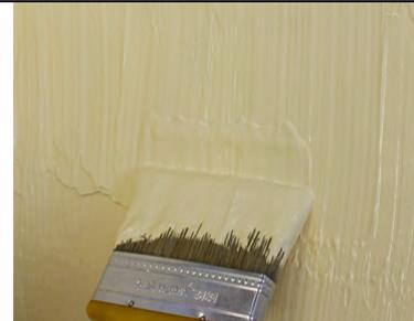
**7.** Apply second coat at correct thickness perpendicular to first.
