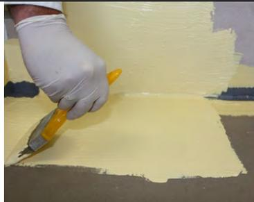
**6.** Apply first coat of membrane at correct thickness across entire section (including full surface of bandage).
