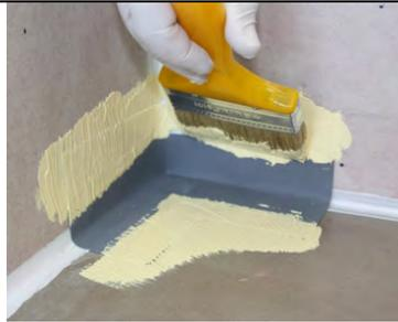
**5.** Secure bandage by applying chosen membrane to open flexible weave.
